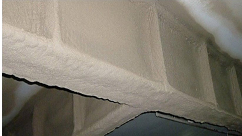
Sprayed-On Fireproofing
