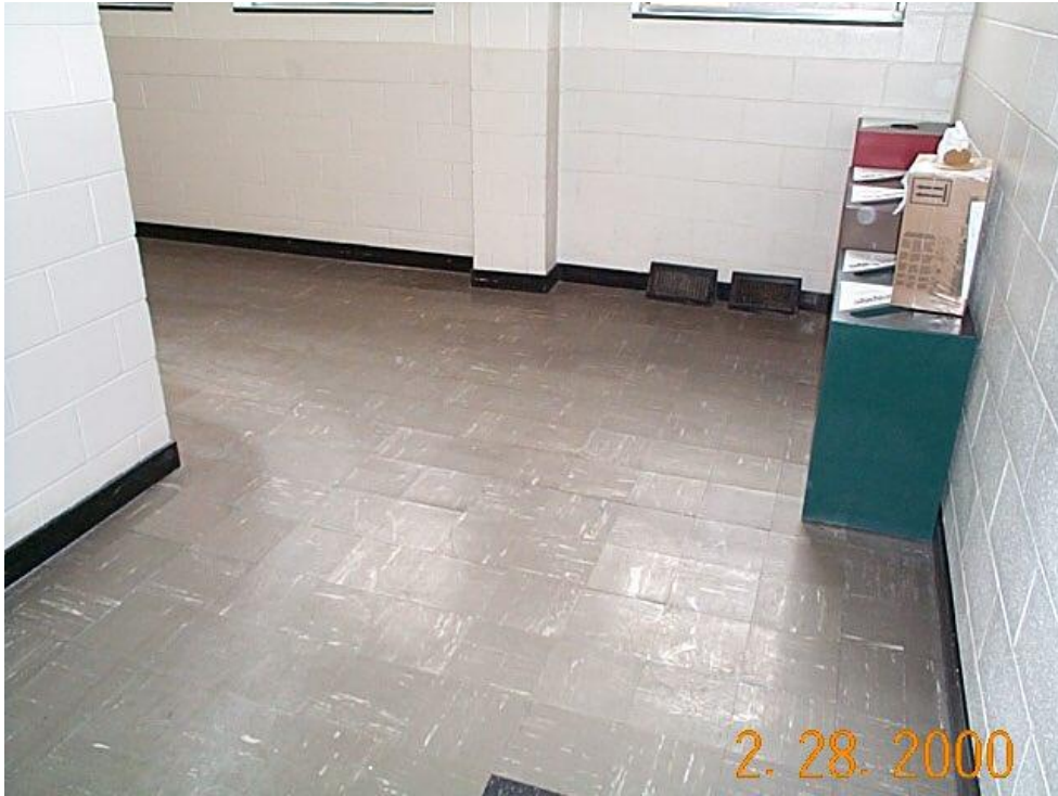
Floor tile and mastic
