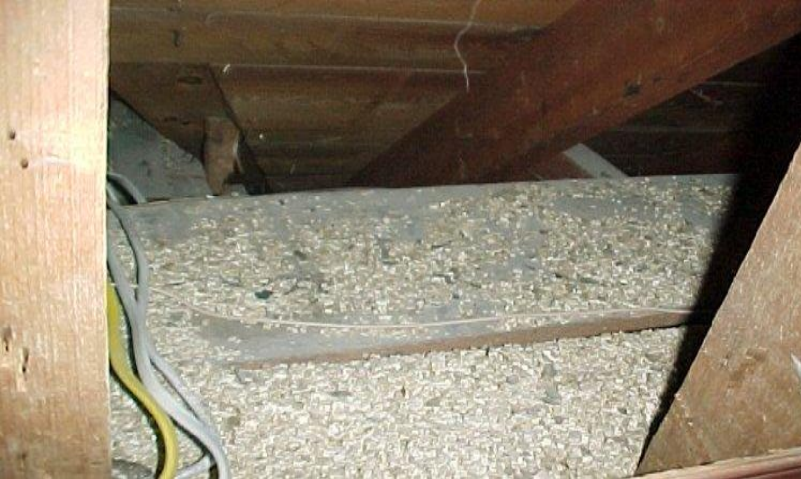
Blown-in Vermiculite insulation in attics
