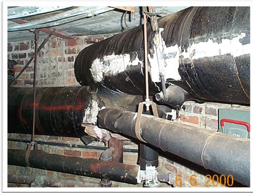
Various types of lagging, coverings and mudded fittings
