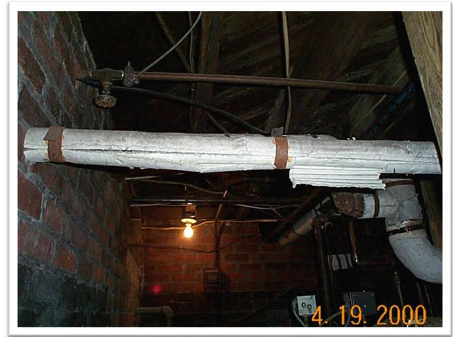
Various types of lagging, coverings and mudded fittings
