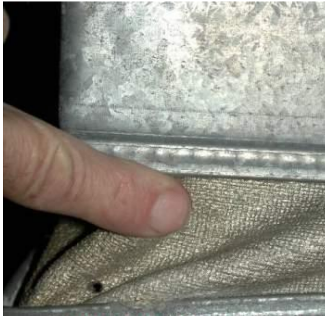
Flexible Duct Connector
